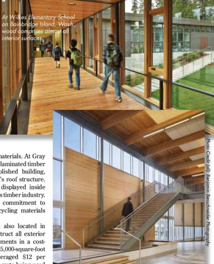
At Gray Middle School in Tacoma, Wash., glue-laminated timber beams were salvaged from a demolished building, sanded and reused in the new school's roof structure.
