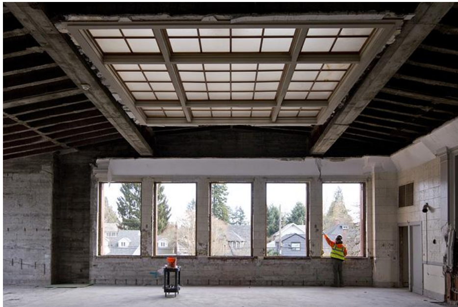
The building has been stripped down to its structural elements; selective demolition and abatement is approximately 80 percent complete.
