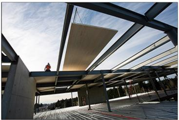
Photo courtesy of KPFF Consulting Engineers [enlarge] Cross-laminated timber was used instead of metal and concrete decking for the roof of this health clinic in Shoreline.
