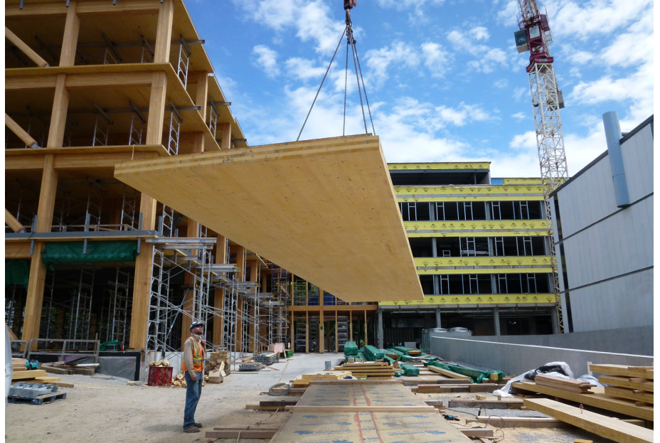
CLT roof panel lifted into place. Image: Structurlam
