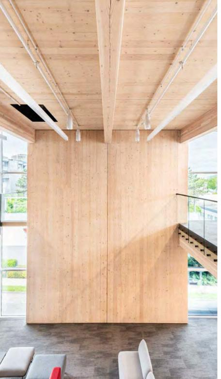
IMAGE: CLT shear wall at Fast + Epp's Vancouver, BC office
