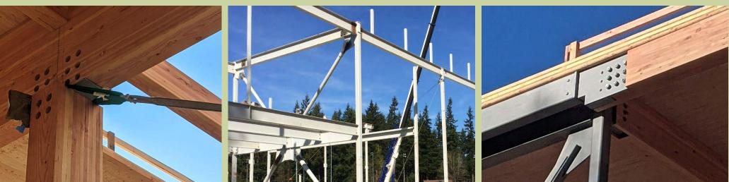
Mass timber post and beam construction with CLT floor deck.
