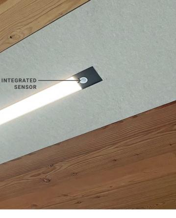
IMAGE, ABOVE: Example of luminaire with embedded controls. The sensor in lighting could include CO2, Temperature, Humidity, Occupancy, Photosensor, Bluetooth beacon, etc.
